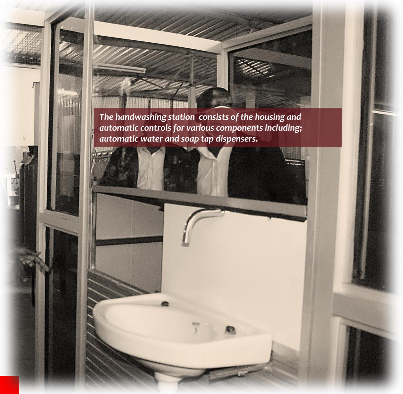
*The handwashing station consists of the housing and automatic controls for various components including; automatic water and soap tap dispensers.*
